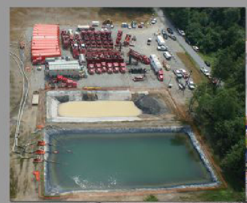
Well pads & impoundments
