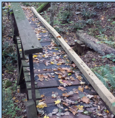
The FOCSP furnishes the Over the Hill Gang with money and materials to make the bridges safer with roofing shingles and fenders
