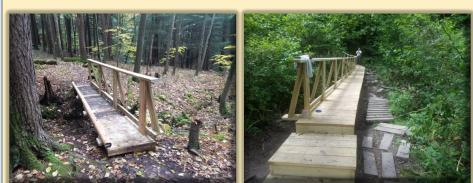
Here The Gang was working on replacing the longboards between the Jersey Bridge and the bike trail. The bridge is elevated and there are steps on either end.
