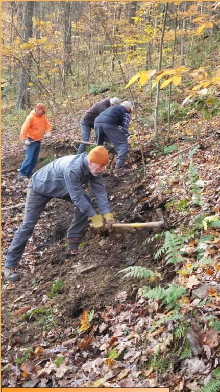
Rebuilding trail that a large, old oak took with it as it fell
